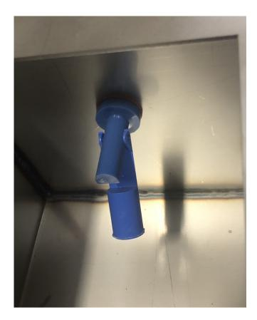
New float switch installed.
