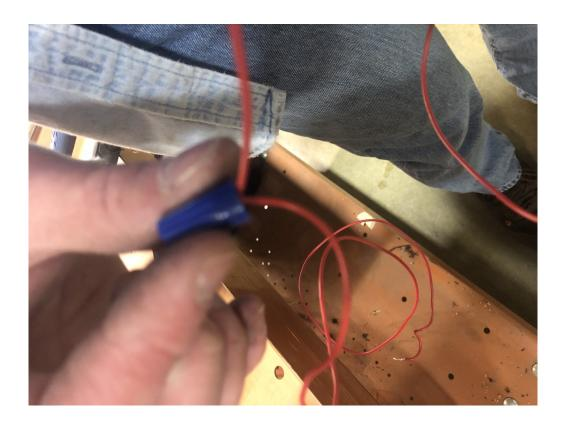
Use wire nuts to connect wires. Replace the electrical box cover using the 7 screws.
